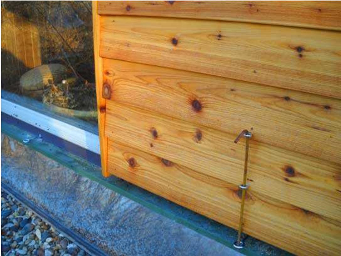
To operate them we simply pull the rod upward, pull the panel out from the wall slightly to allow the side-mounted 1-by-4's to slip past the windows that they partly surround, slide the unit sideways, then lock it down in the other position. During extreme cold we may have to be careful to avoid sudden thermal shock to the windows by opening the panels rather slowly.
