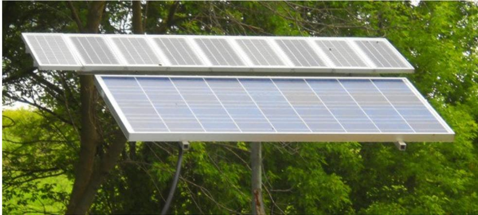
I started with 8 panels, wiring them to a switch-box that allowed the panels to either charge the Honda at a very high voltage that matched its battery pack, or could switch it to trickle-charge both our 12-volt mower and our old 36-volt G.E. Elec-Trak electric garden tractor. Here is the wiring diagram:
